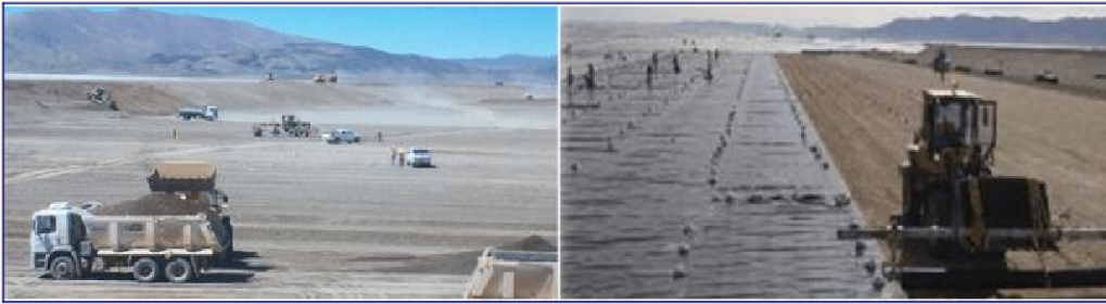
New carbonation plant & soda ash facility footings for Olaroz Stage 2
