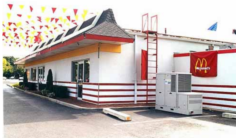
McDonald's restaurant in North Babylon (NY) partially powered by a fuel cell (Source: LIPA)
