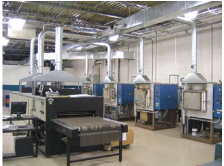
HydroGen Corporation manufacturing 400 kW PAFC modules - the building blocks of its 2 MW commercial system - at its plant in Versailles, Pennsylvania.
