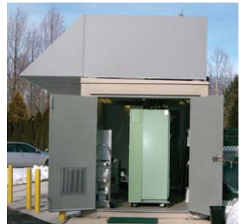
Ztek 25 kW Solid Oxide Fuel Cell with 4 ton HVAC on Roof Top
