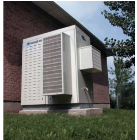
Hydrogenics' HyPM 8-XR DC Backup Power System deployed at a Bell Canada telecommunications site with Emerson Network Power
