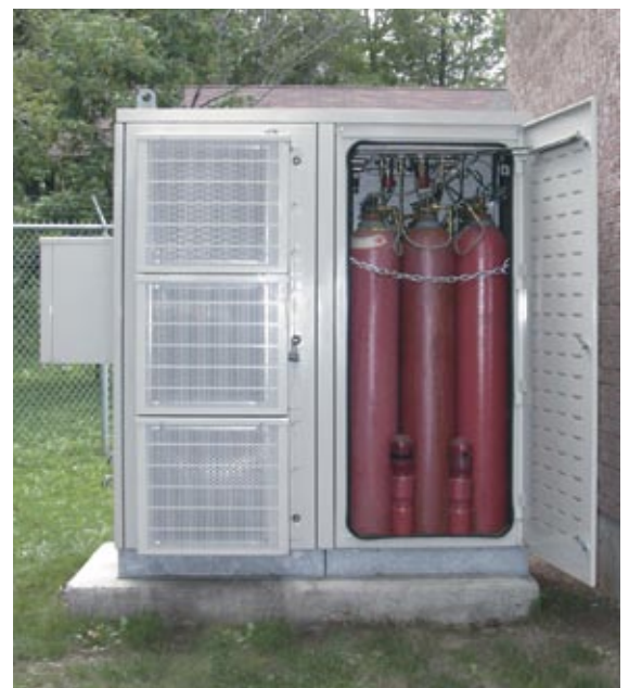
HyPM XR DC Backup Power System with fuel storage
